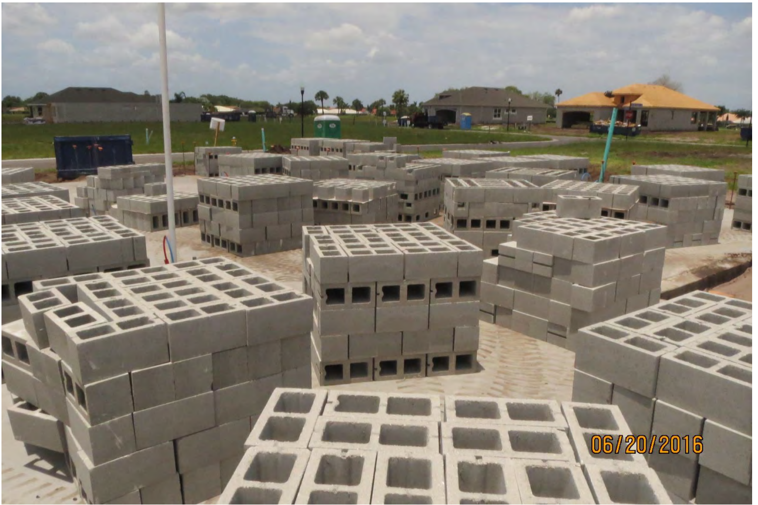
“Bond beam” or open-top blocks shown below:
