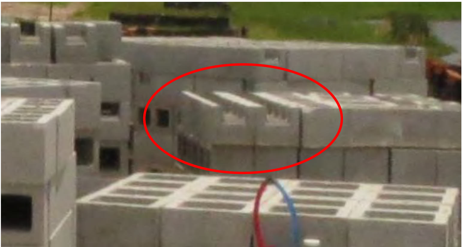
“Bond beam” or open-top blocks shown below:
